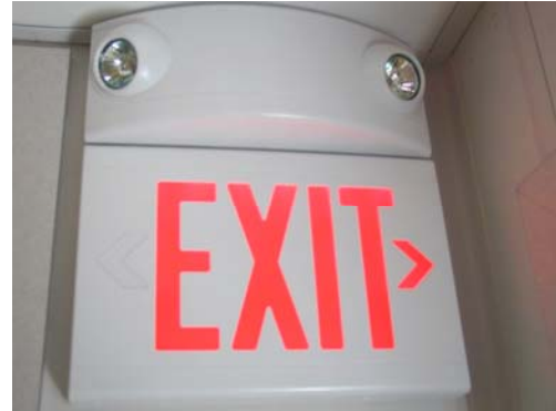
Figure 21: Emergency Lighting
